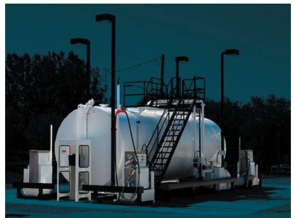
Installation shown: Weather booth used with a "Fuel Stop" Unattended CardLock Fueling Station
